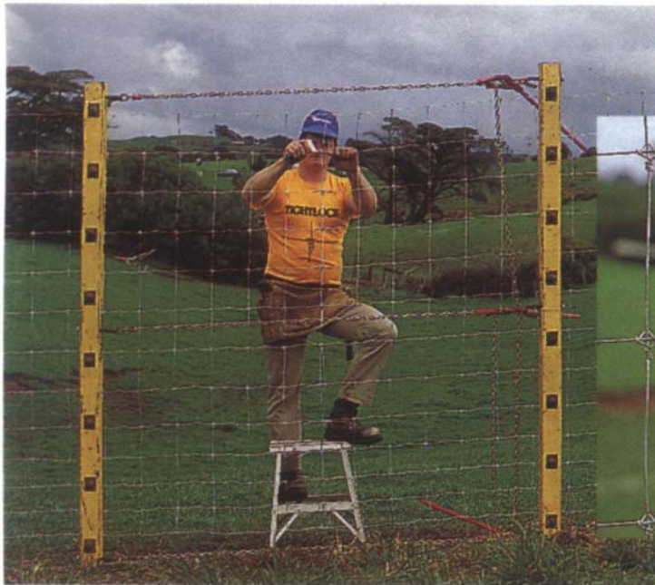
Splicing the netting together (un-tensioned between strainer boards)
