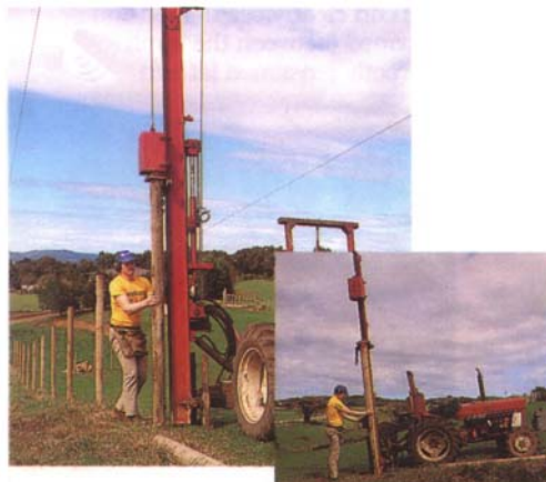
Laying out & posting
