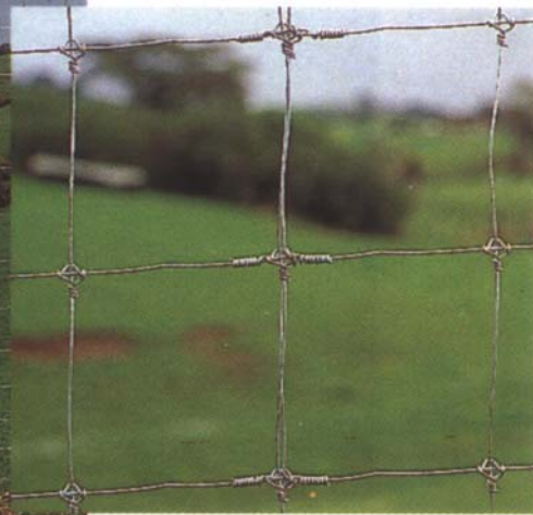
Each knot is overlapped and tied off
